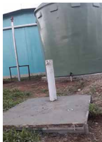
A tap stand and tank constructed for the project - yet to be fenced off from animals
